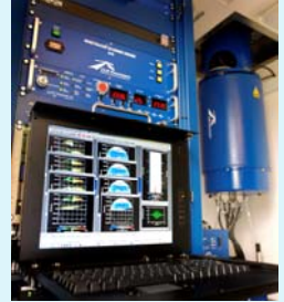
View inside the Lidar shelter: electronics rack with operator GUI (left) and laser unit (right)
