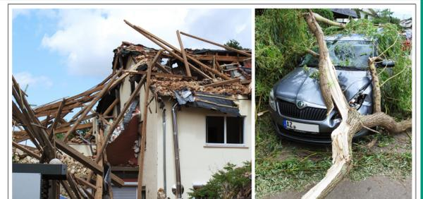
Fig. 1: Losses associated with a microburst event in Framersheim (Rhineland-Palatinate, Germany) on 7<sup>th</sup> June 2015 (© Susanna Mohr).
